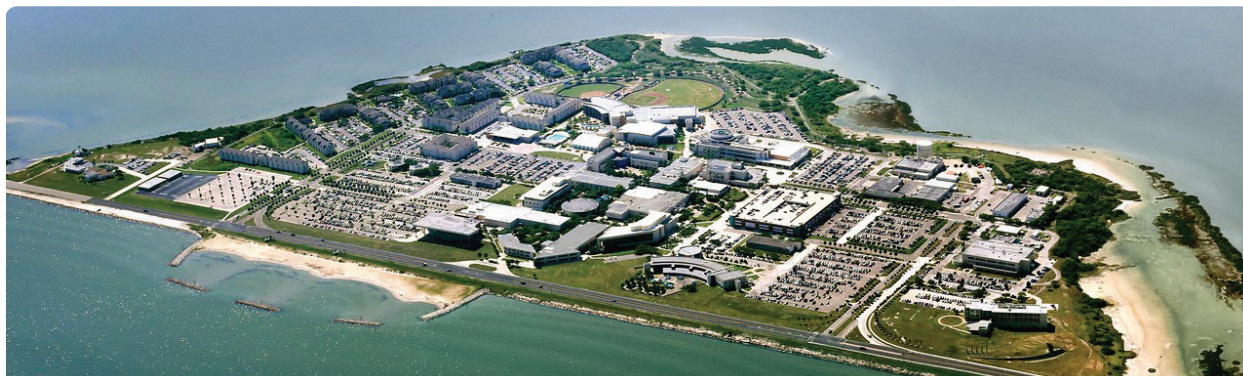
Aerial Image of Texas A&M - Corpus Christi
