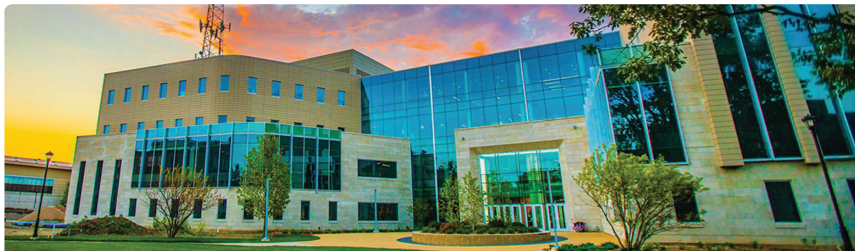
Business and Engineering Convergence Center
